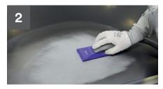
Hand block or machine sand the repair area using 3M™ Hookit™ Abrasive Sheet P320.t
