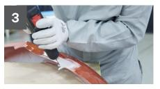
Drill several holes of 3 – 6mm in diameter in the remaining part of the tab to increase the strength of the repair.
