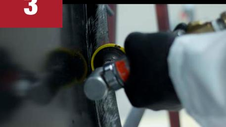
Clean with **SEM Solve** or **XXX Universal Surface Cleaner**. Grind mating flanges with a P36 grit grinding disc at low speed for aggressive grind mark. Remove any adhesive or protective coatings.
